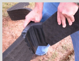
Inserting into fitting/tape
