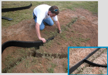
Installing J-DRain SWD-6 into shallow trenches
