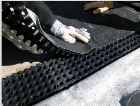
Figure 1. J-DRain GRS core has inter-locking dimples
