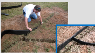
INSTALLING J-DRain GRS
