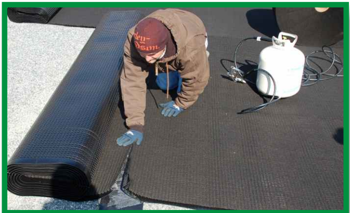
Butt Joint Detail: Step 2
