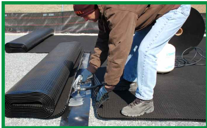
Butt Joint Detail: Step 1
