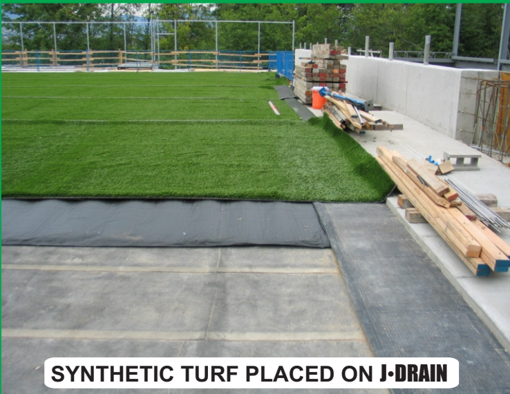
J-DRAIN MVP-12 FOR LATERAL DRAINAGE
