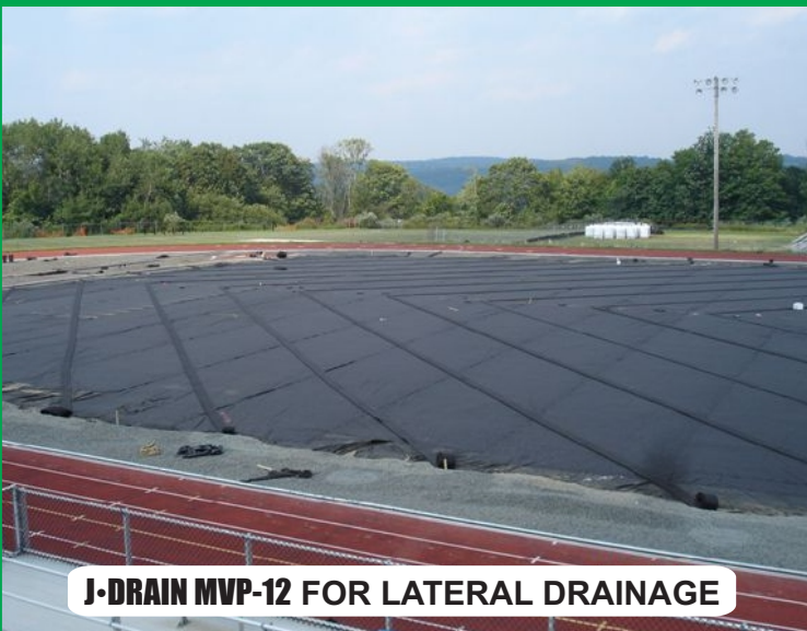
DRAINAGE LATERALS INTO SIDELINE TRENCH
