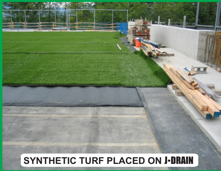
J-DRAIN MVP-12 FOR LATERAL DRAINAGE
