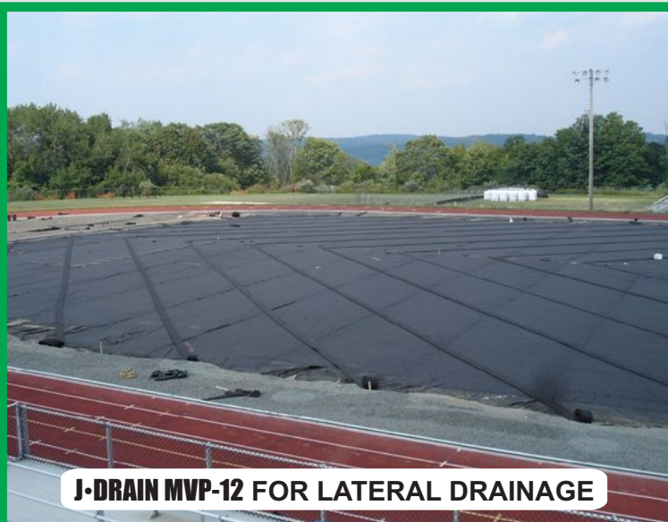
DRAINAGE LATERALS INTO SIDELINE TRENCH
