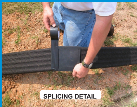
INSTALL AND TAPE FITTINGS
